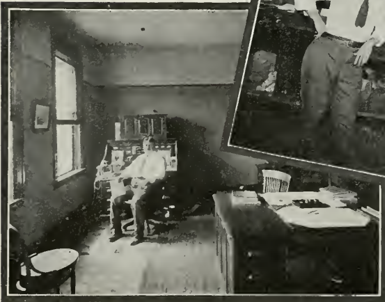
OFFICES OF PATTERSON COAL AND SUPPLY COMPANY
